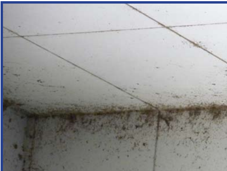
BEFORE: Emergency Room Exit
