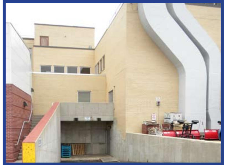
AFTER: Loading Dock
