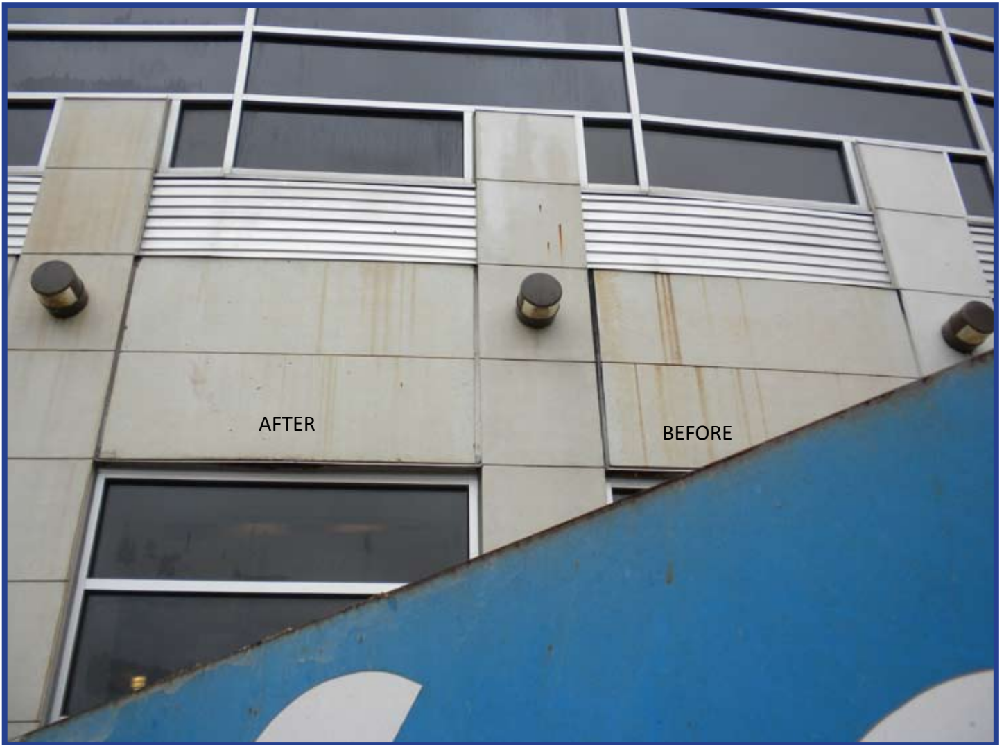
Diminished rust stains on delicate stone surface of hospital.
