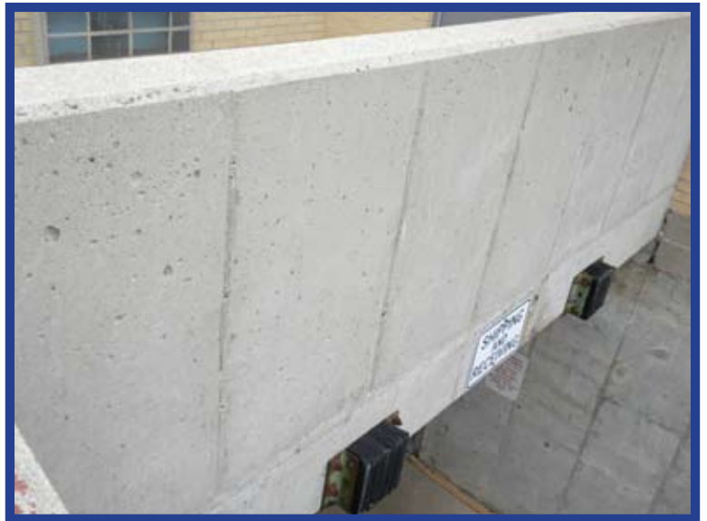
AFTER: Loading Dock
