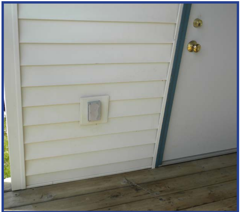
DECK & SIDING AFTER CLEANING
