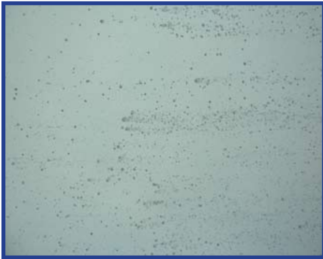
Closeup - Mildew on door backside - Before
