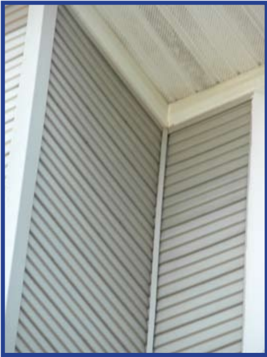
Front corner cleaned of debris
