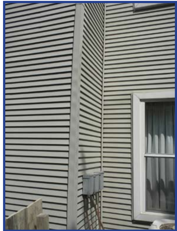
Corner Cleaned - Backside
