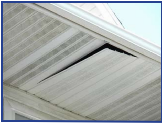
Repair Before - No Charge
