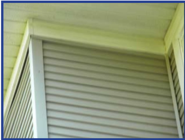
All debris removed from backside. Upper corner - buildup removed.
