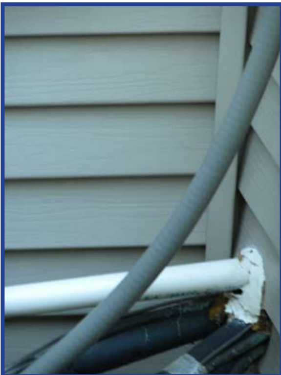
All lower corners cleaned - backside by air conditioners
