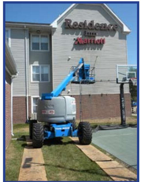
Plywood laid as agreed
