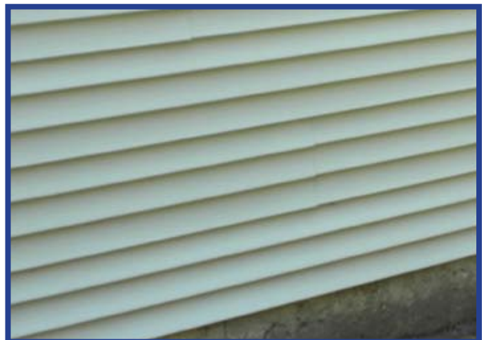
Siding cleaned - After
